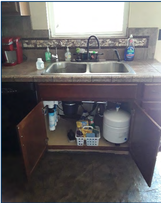
POU device units installed under the kitchen sink of the Fleinshauer household.
