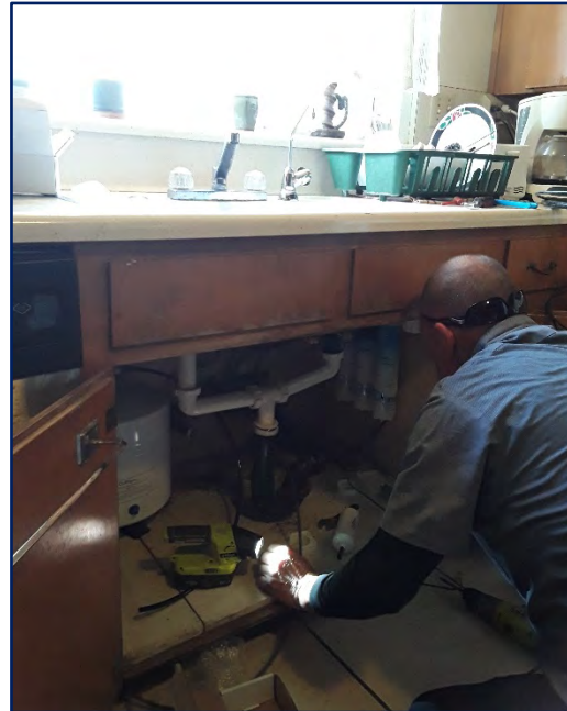
Culligan staff member installing a POU device at the Eaton household.
